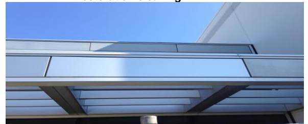
Clear anodized aluminum panels cleaned, and center panel sealed
