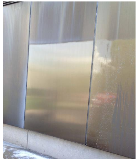
Dark bronze duranodic aluminum-machine polished with our proprietary four step process removes 40 years of oxidation.
