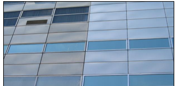
Years of oxidation removed with safe acid free restoration cleaning.
